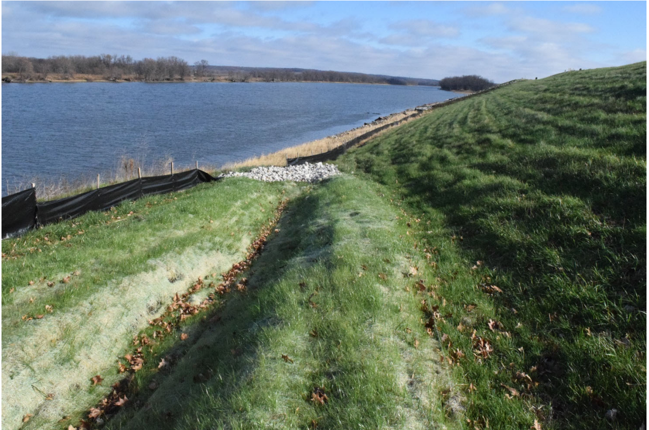
North side exterior
