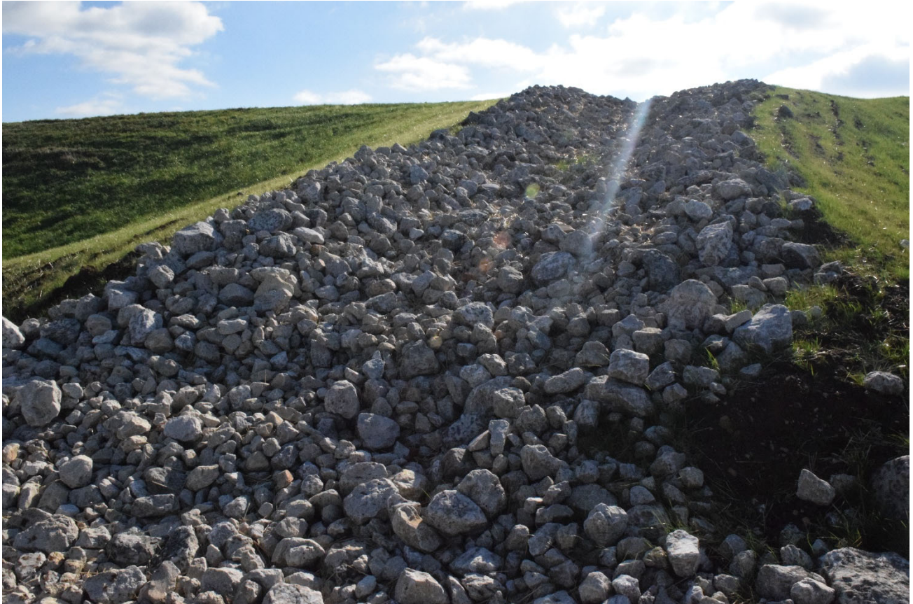
North side let down structure - typical
