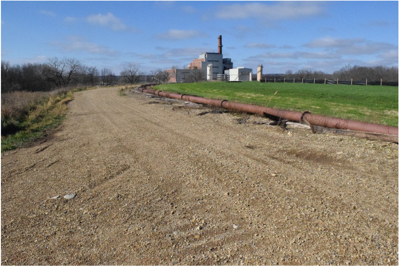
West side crest – west interior filled
