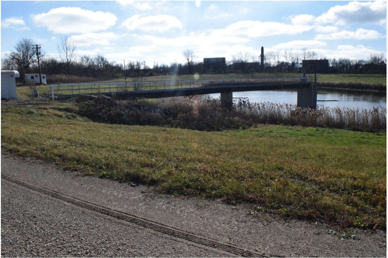
Secondary pond outlet structure and bridge
